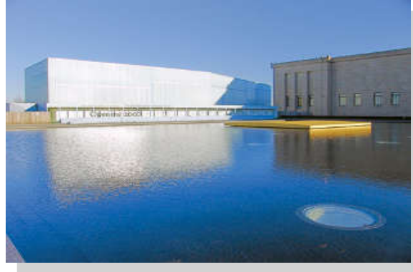
The Nelson-Atkins Museum of Art Bloch Building Expansion / Renovations 1999 - 2007
